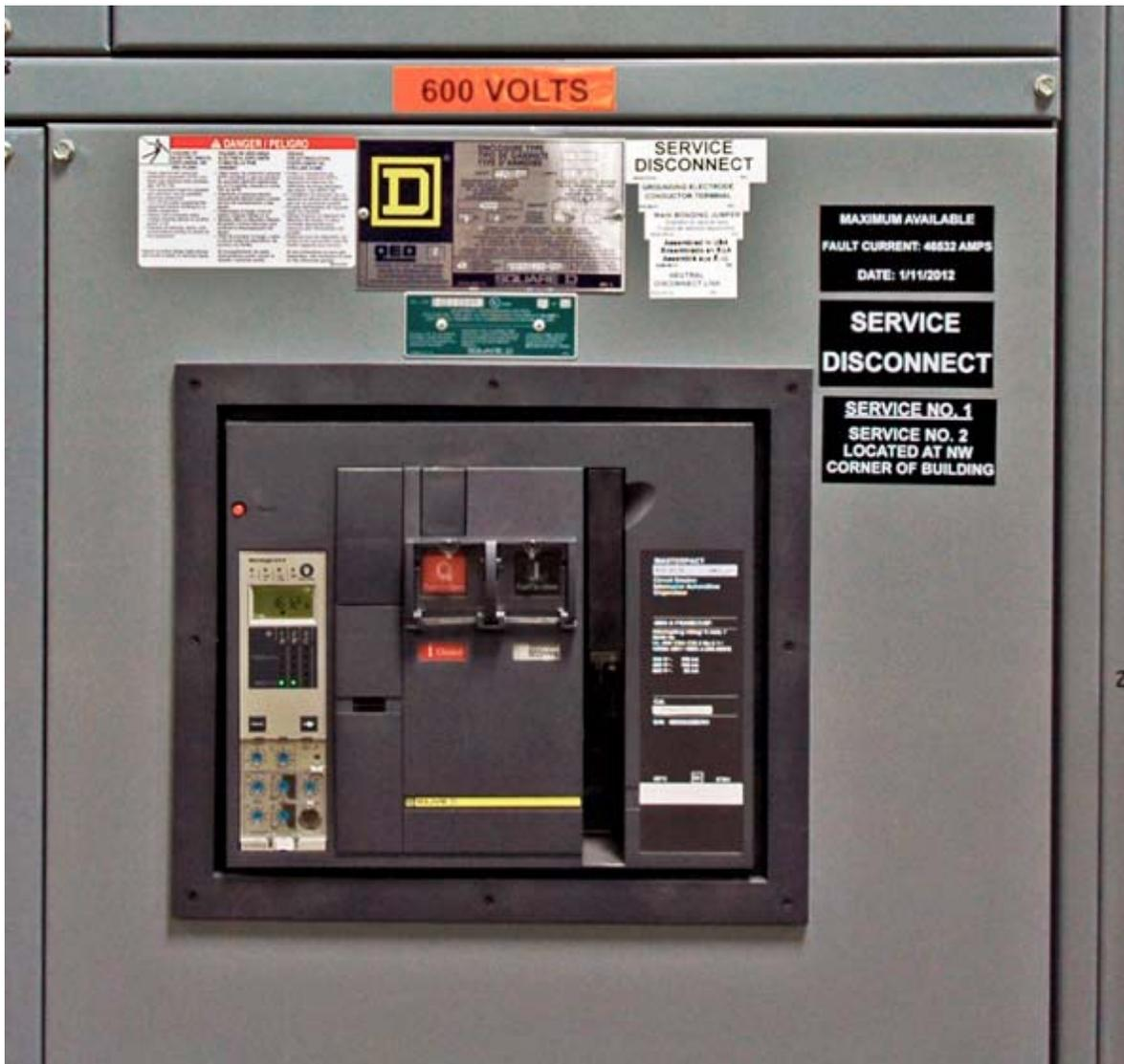
Photo 1. This image shows labels provided by the equipment manufacturer and those field marked by the installer. Note how the labels indicate system voltage and maximum fault current, as well as identify the equipment as a service disconnect. Per ANSI Z535.4, Art. 7.3 and Art. 8.1.2, informational labels like these can be made with white text on a black background or black text on a white background. Always follow the requirements of ANSI Z535 for designing your field-marked labels.
