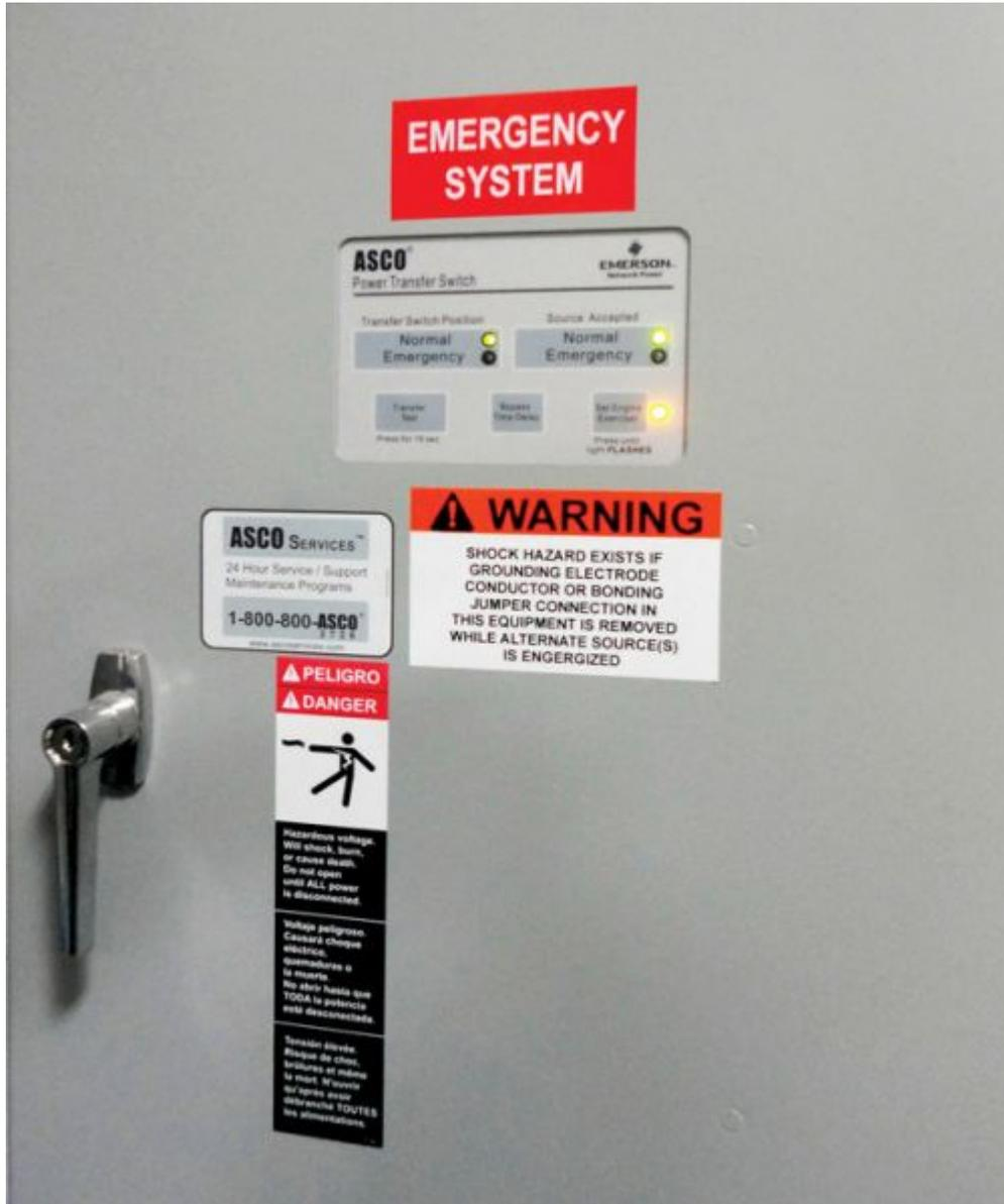
Photo 3. This transfer switch shows examples of how both labels are implemented in an end-user application.
