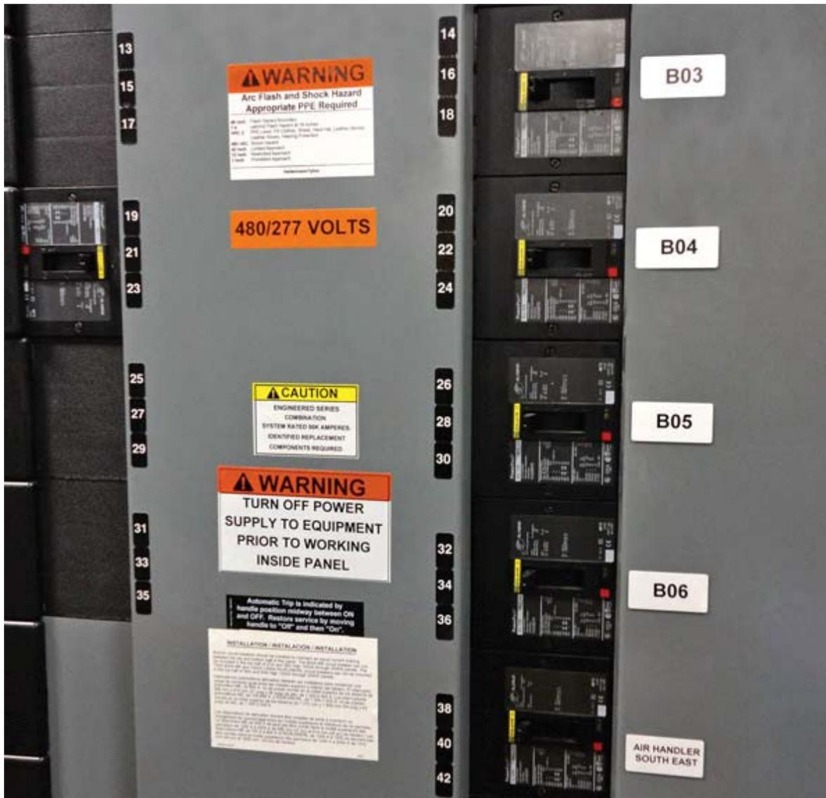
Photo 2. This switchboard is marked with an arc flash label, voltage indicator, and an isolating equipment label. Note that the phases on every circuit are marked, and a separate label identifies each circuit and its intended purpose.
