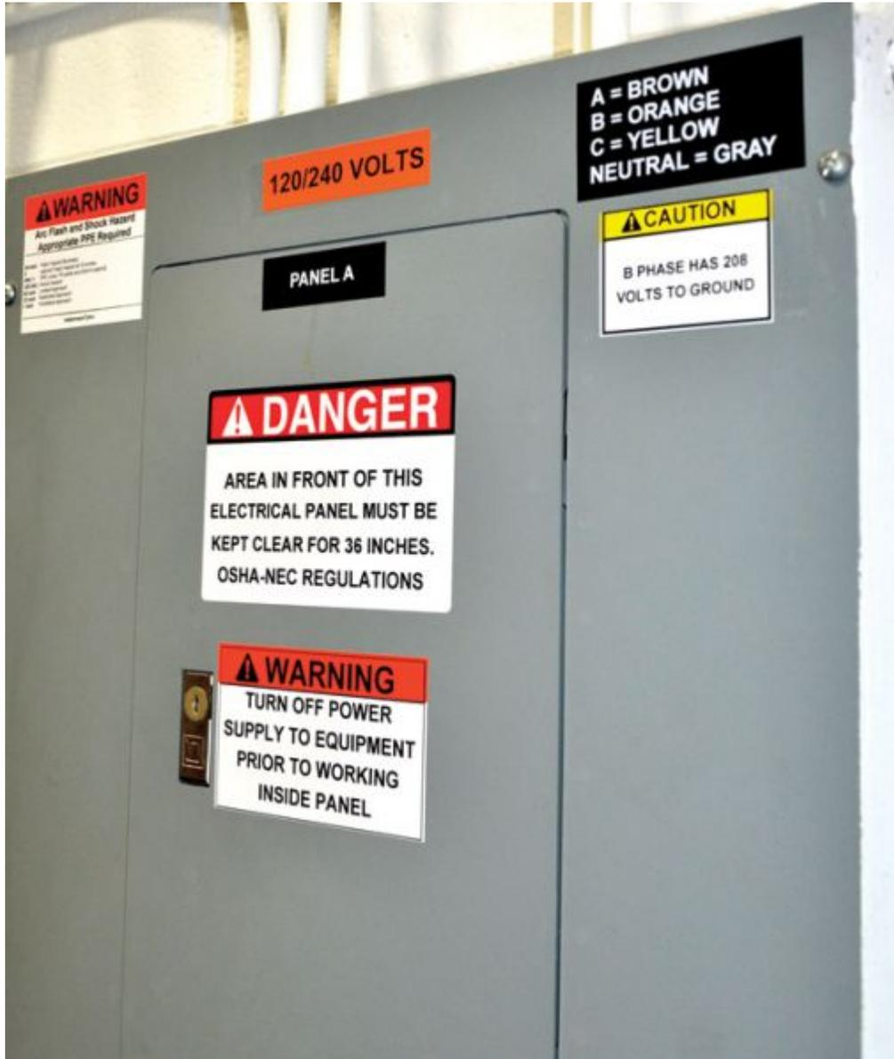
Photo 4. This panel shows all the appropriate labeling as required by the NEC and NFPA 70E, per ANSI Z535 label design formats. Note how the phases are marked in this example.
