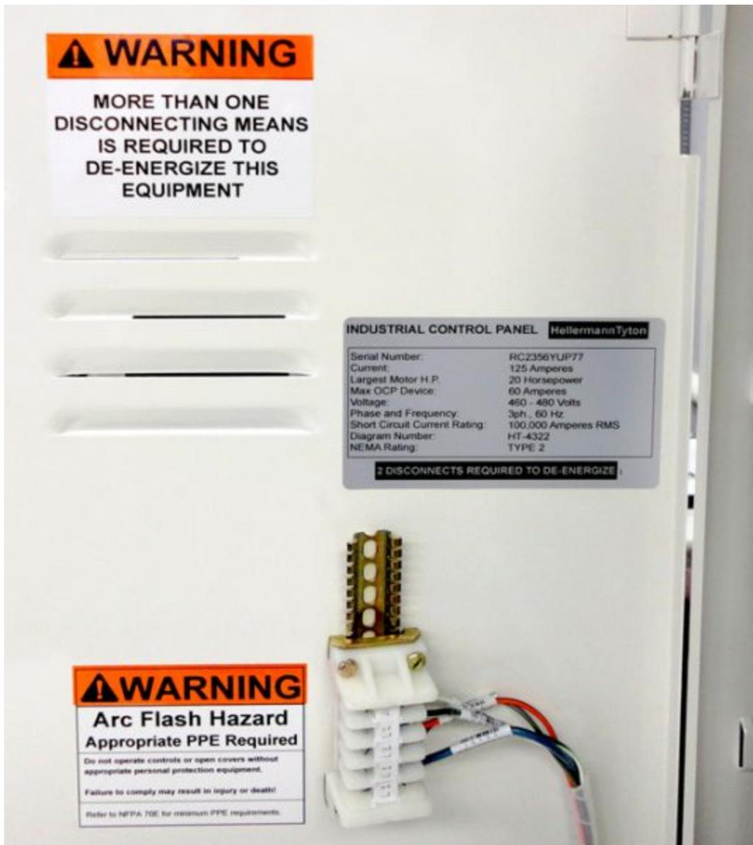
Photo 1. Wires are typically marked with self-laminating vinyl labels or printable heat shrink tubing. Relays and ducting can be identified if specified and relevant to the application. A rating label is shown marked per NEC 409.110(1), (2), (3) and (4) or NEC 408.58 or OSHA 1910.303(e).
